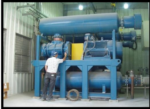
A positive displacement blower is the most common motive air source for the pneumatic transport and fluidization of dry bulk materials.
