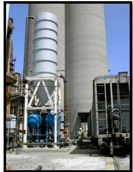
Vacuum unloading of a Railcar
