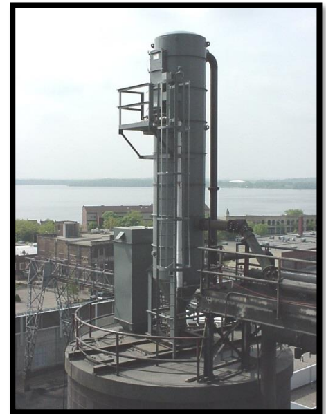
Silo Roof mounted Collector Filter
