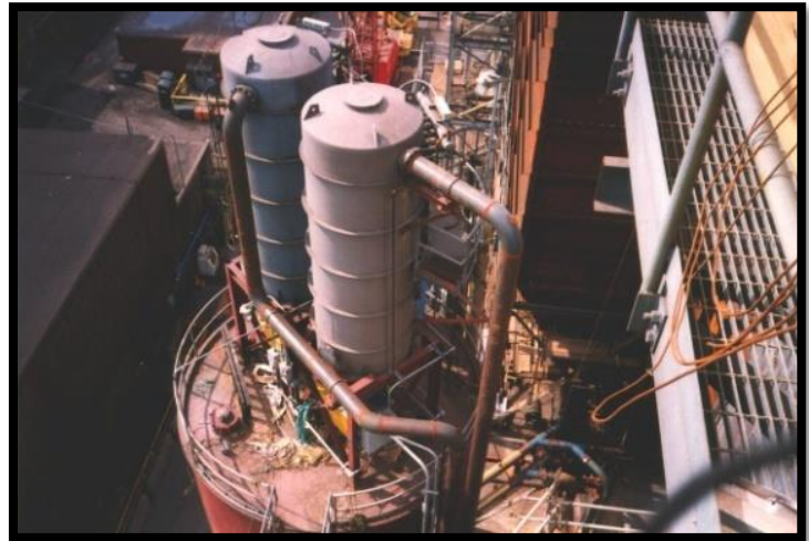
Vacuum Collector/Filters on a silo roof
